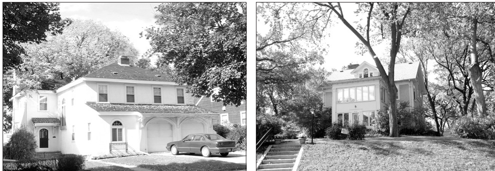
MAC's sound insulation construction costs for these two homes exceeded $120,000 each.
