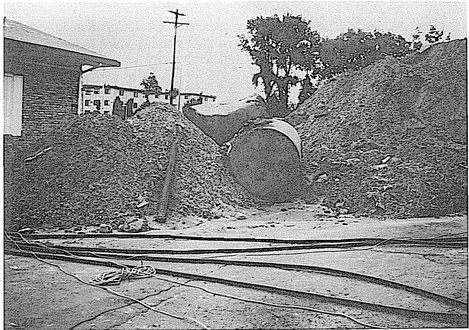
Old, leaky petroleum storage tanks with piles of clean and contaminated soil.
