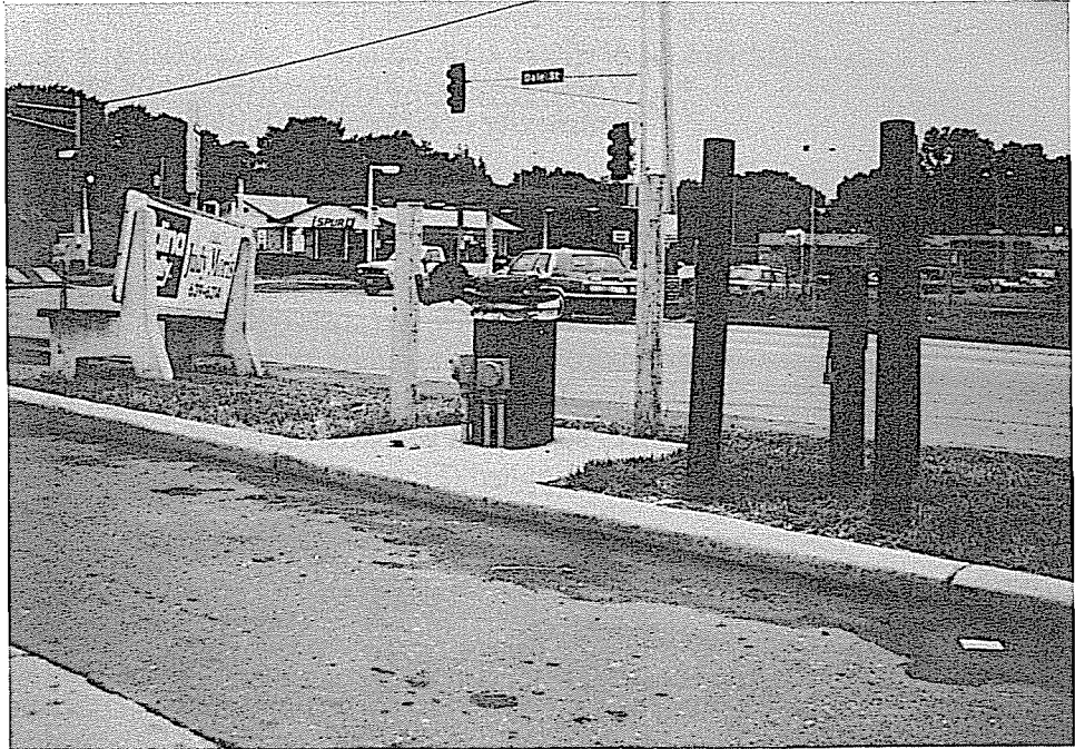
Monitoring well encircled by taller bumper posts at right with recovery well for water treatment at center.
