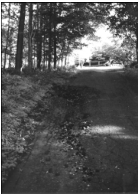
There are some signs of deterioration, such as eroded or flooded trails, in some parks.
