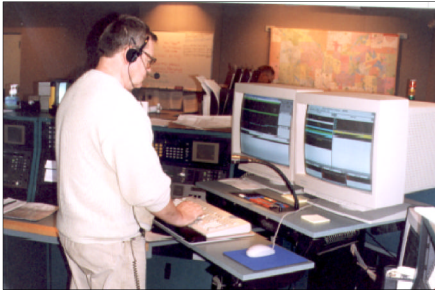
Height-adjustable console accommodates different dispatchers
